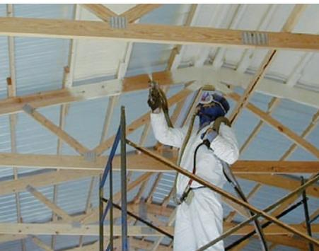
BaySeal™ is applied to exterior walls and roofs as a heated liquid which then quickly expands, completely filling every open
